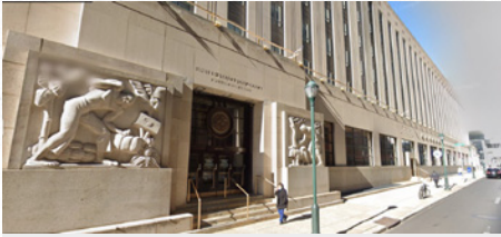
Today: View from 9 th Street – Post Office
